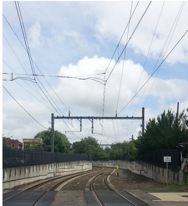
Figure 2 NJ Transit Catenary System
